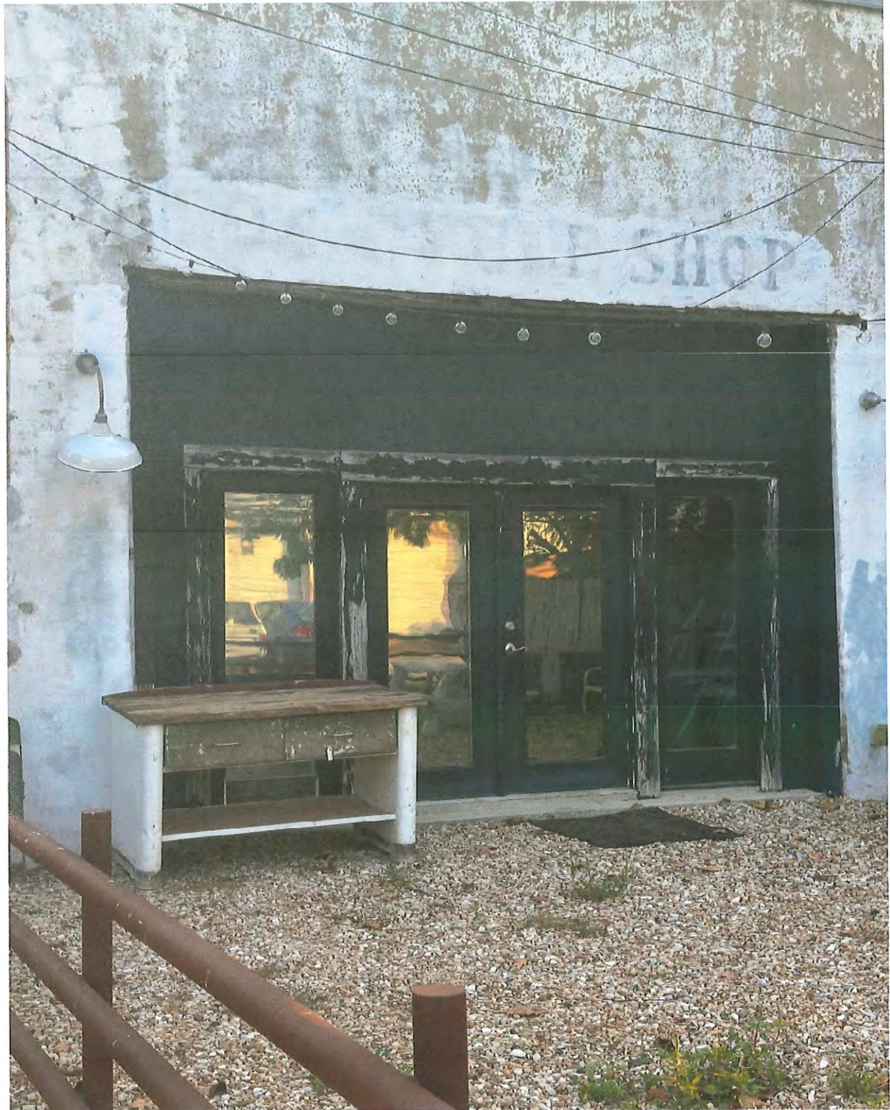
Figure 5.1. Rear Door, Framing, & Stucco
